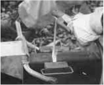
Joining of rails by mould welding: OK 74.78.
